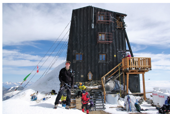
Figure 13. The building of the Capanna Regina Margherita hut
