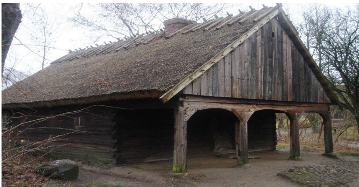
Photo 1. Gburska cottage from Wdzydze Tucholskie with a full-top three-bay arcade, transferred to the Kashubian Museum in Wdzydze Kiszewskie (photo by Patrycja Essing)
