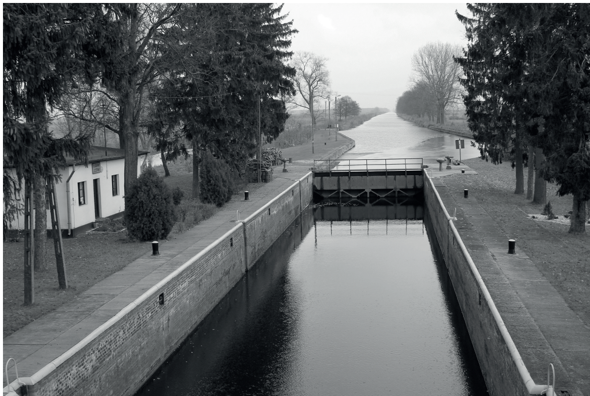
Figure 2. Józefinki Lock and the view on the Bydgoszcz Canal eastwards (photo made by the author, 2017)
